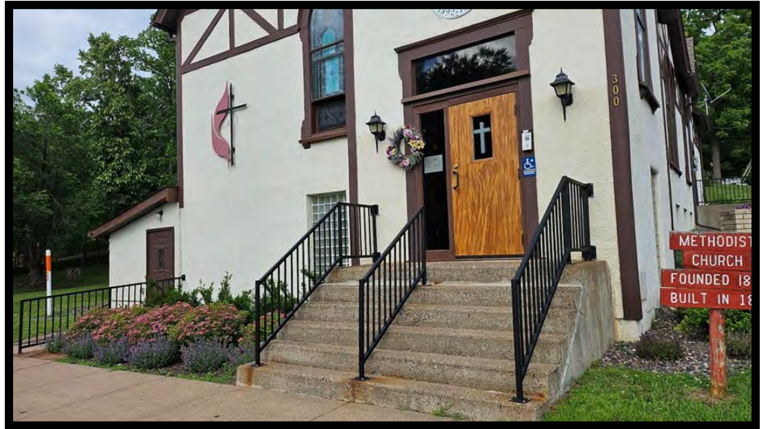
6-18-2026, New Railing installed at St. Croix Falls UMC
